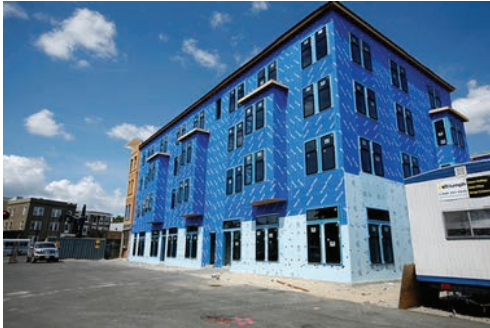
"Peel & stick" air barrier applied to rigid insulation
