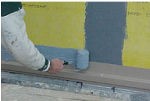
Sealing the air barrier connections
