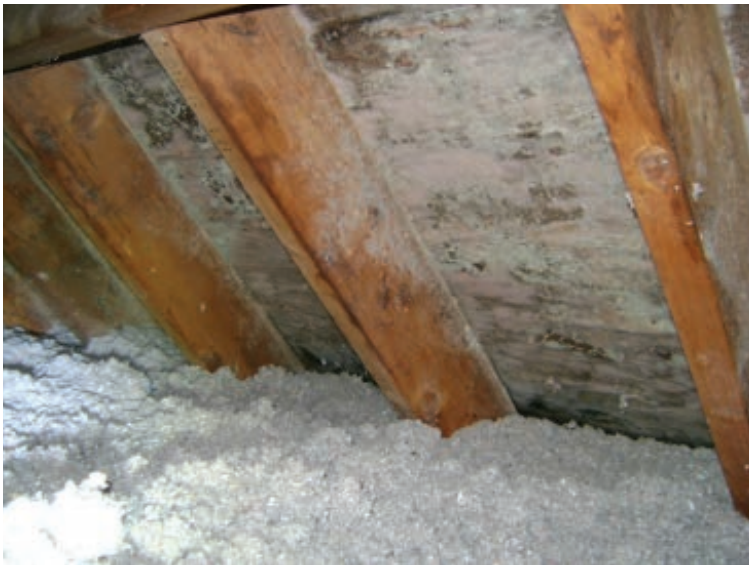
Above depicts microbial growth due to uncontrolled moisture-filled airflow in an attic
