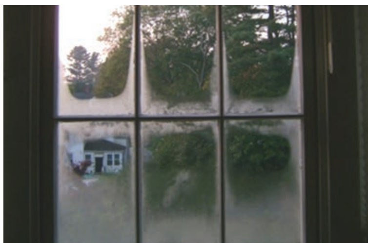
An example of excess interior moisture, condensing on a cooler window surface
