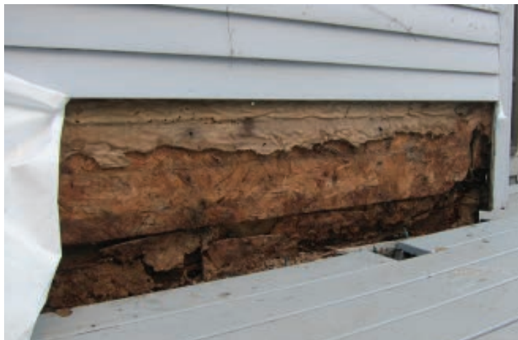
Image shows water damage due to poor flashing and/or drainage plane technique
